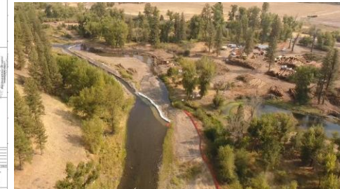
Bird Track Springs Construction September 2018
